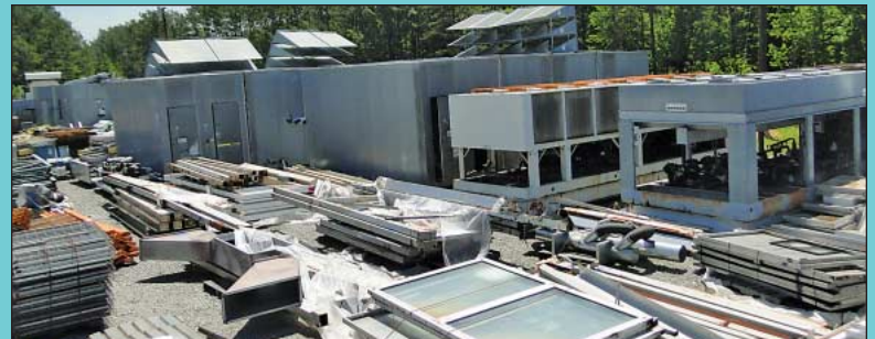
Large Paint Line Including Paint Booth and Oven Components, Air Make-Up Units, Chillers, Duct Work, and Exhaust Fans
