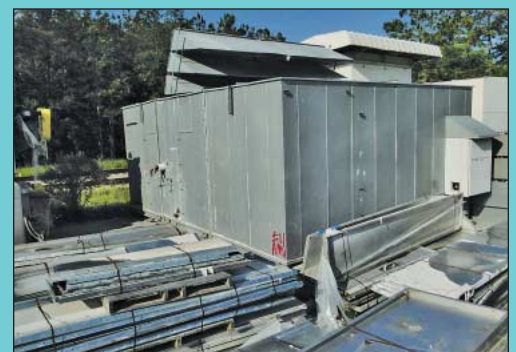
Close-Up View (1 of 5) Air Make-Up Units
