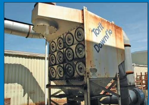
30 HP Torit Donaldson Downflo Model T3-24 Cartridge Type Dust Collector
