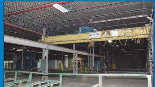
7-1/2 Ton X 35' Approx. Span Progressive Double Girder Top Running Overhead Bridge Crane
