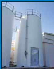
(4) 12' Dia. X 24' High A.O. Smith Welded Steel Material Storage Silos
