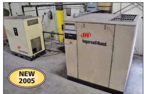
100 HP Ingersoll Rand Model SSR-EP100 Rotary Screw Cabinet Enclosed Air Compressor
