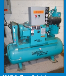
25 HP Sullivan Palatek Horizontal Tank Air Cooled Rotary Screw Air Compressor
