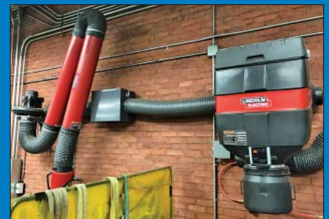
(3) Lincoln STATFlex 400-MS Fume Collectors
