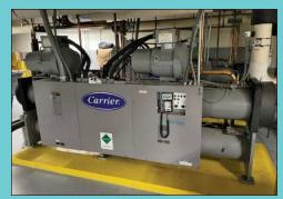
(4) 114 Ton Trane Model 30HXA116RY-640 High-Efficiency Indoor Liquid Screw Chillers
