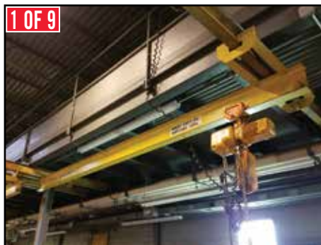
1 OF 9 (9) 1-1/2 Ton x 18' Underhung Single Girder Bridge Cranes
