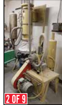
(9) Vacuum Pumps w/ Inline Resin / Dust Filters
