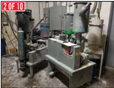
(10) Vacuum Pumps w/ Dust Waste Canisters
