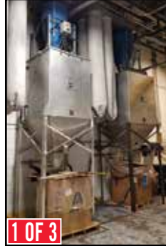
(3) Towers w/WHITLOCK Vacuum Locks
