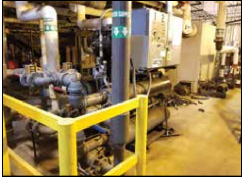
AEC Chiller System
