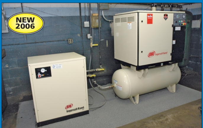
30HP Ingersoll Rand Model SSR-UP6-150 Air Compressor w/ Air Dryer
