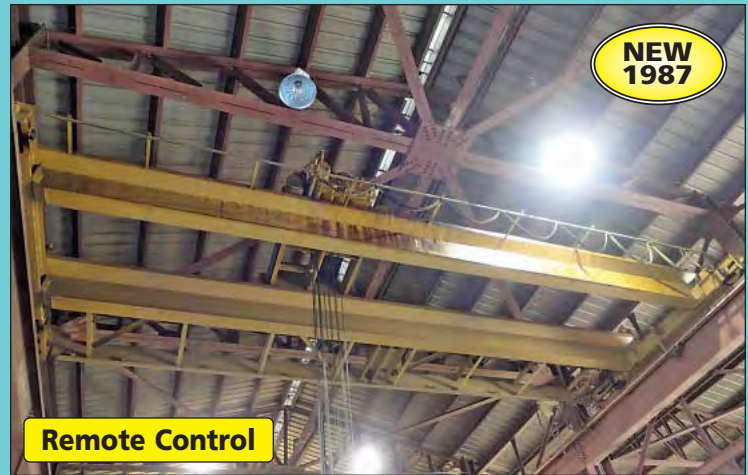
15 Ton X 40' Approx. Span Pelham Double Girder Top Running Overhead Bridge Crane
