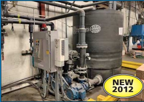
1,500 Gallon Advantage Engineering Model TTKC-1500-3P 3-Pump Skid Mounted Poly Insulated Chilled Water Pump Tank
