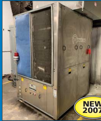
25 Ton Advantage Engineering Model C-25APT-10HBX Portable Air Condensed Chiller
