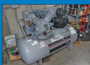
10HP Ingersoll Rand Model 2454F10 2-Stage Horizontal Tank Rotary Screw Air Compressor
