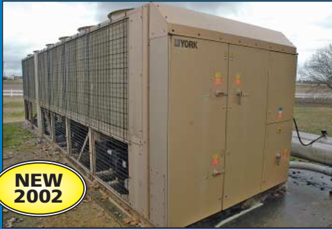
(2) 270 Ton York Model YCAS0270EC46XFADB Central Water Chillers
