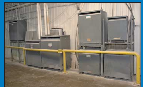
(24) Transformers From 75 to 250 KVA Manufacturers Include Federal Pacific, GE, Cutler Hammer and Square D
