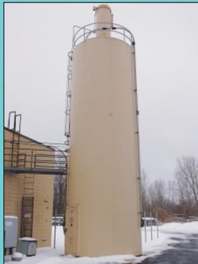
12' Dia. X 36' High Imperial Calumet Model 60-40-12 X 36 Welded Steel Material Storage Silo
