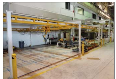
(3) 2,000 Lb. X 24' Approx. Span X 36' Approx. Long Spanco Free Standing Overhead Crane Systems
