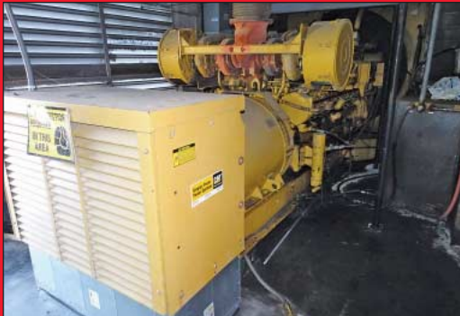
1,550 KVA Caterpillar Model 3516 Diesel Generator Set
