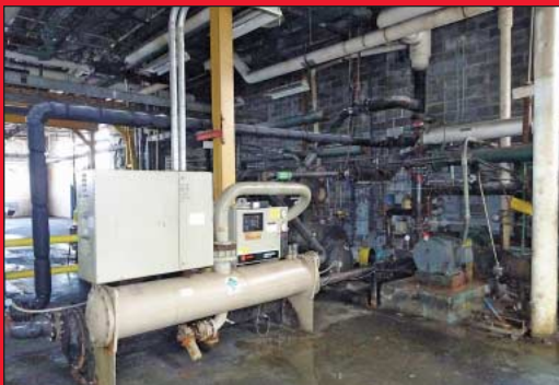
215 Ton Trane Model RTHA215A0 Centravac Series R Water Condensed Rotary Compressor Central Chiller
