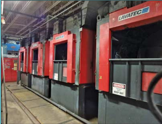
(6) 200 LB Lavatec Model TT745GU Gas Fired Batch Dryers
