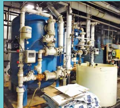
(2) Water Softening Tanks with Controls
