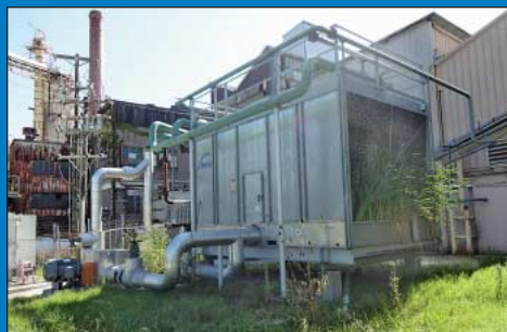
Marley Model NC Class Cooling Tower
