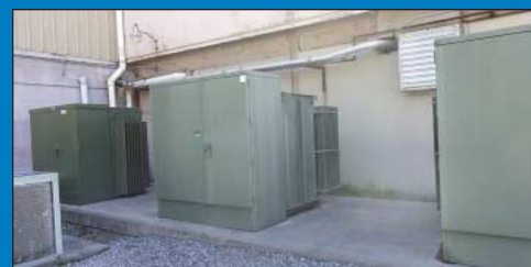
(4) 1,000 KVA Howard Industries & Ermco Transformers
