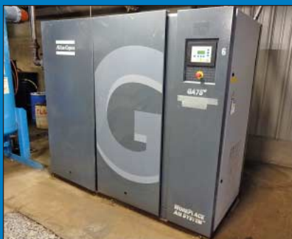
(2) 75 HP Atlas Copco Model GA75+ Air Compressor
