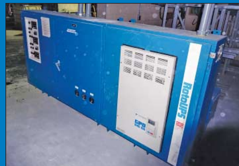
International Computer Power Model RU100K633-HH-AB-MB-RA Uninterruptible Power Supply (Roto UPS)
