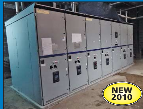
7-Section Cutler - Hammer VACCLAD-W Metal-Clad Switchgear Station
