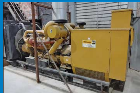
750 KW Caterpillar Model 3412 Generator
