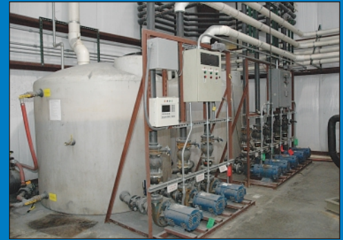
(2) 2,100 Gallon Plastic Tanks w/ Pumps
