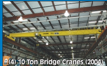
(4) 10 Ton Bridge Cranes (2004)
