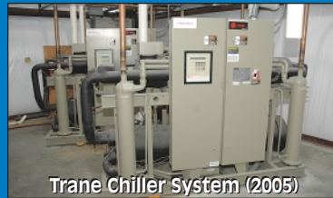
Trane Chiller System (2005)
