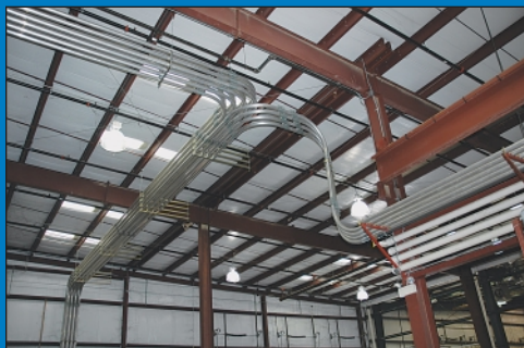
Approx. 4800' - 3" Dia. Aluminum Material Delivery Piping
