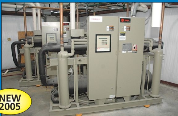
(2) Trane Model RTUA-1004-XG01-R3C0-FNY Air Cooled Central Chiller Systems
