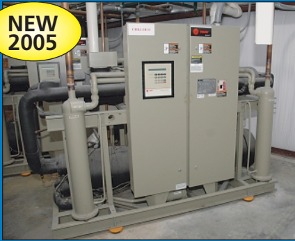
(2) Trane Model RTUA-1004-XG01-R3C0-FNY Air Cooled Central Chiller Systems
