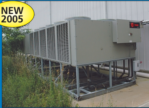
(2) Trane Model RTCA-10040G00-A300GKN Remote Outdoor Evaporation Units
