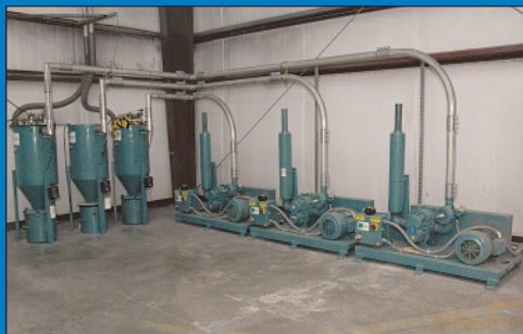
Partial View Una-Dyn Central Material Loading System
