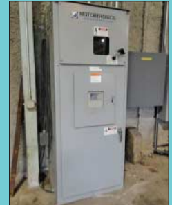
4,160 Volt / 200A Motortronics Solid State AC Motor Control Center at 1,250 HP Nominal
