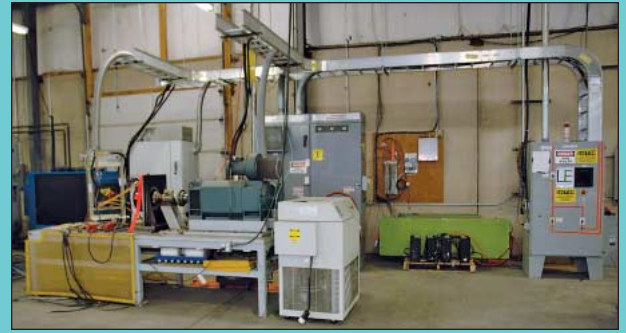
300 HP Dynamometer Test Stand w/ Motor, Control, Chiller and Related
