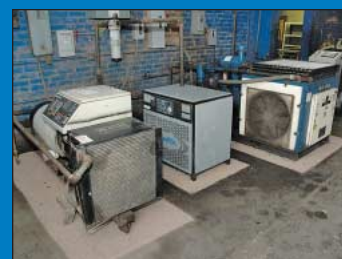
Bank View of 50 H.P. and 25 H.P. Air Compressors and Air Dryer
