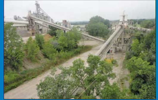
Partial View Large Quantity of Aggregate Conveyors To 60" Wide and 310' Long
