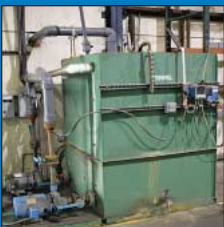
Cooling Tower System Including Advantage Pump Tank
