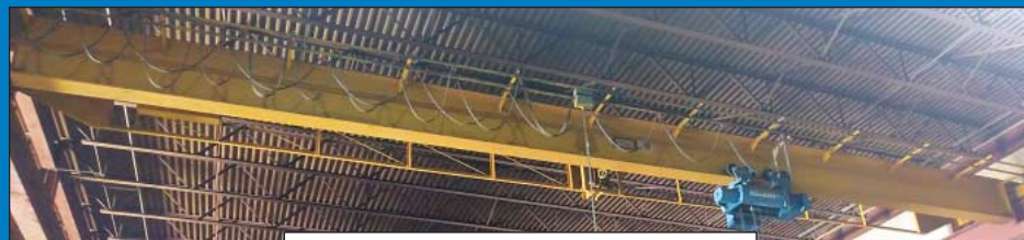
(2) 10 Ton X 60' Approx. Overhead Bridge Cranes
