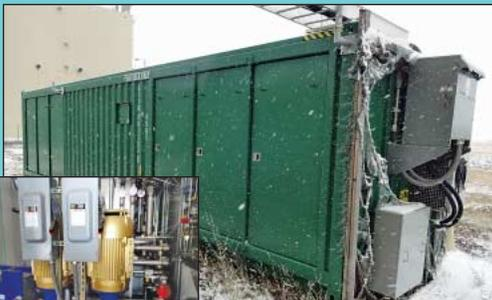
Containerized Chilled Water System
