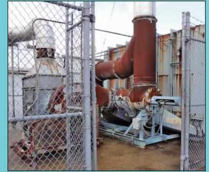
Tellkamp Model Roxidizer Paint Fume Thermal Oxidizer Burn-Off System
