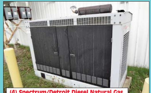
**(4) Spectrum/Detroit Diesel Natural Gas Generators Up to 81 KW (New as 2002)**
