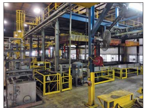
Large E-Coat Line Consisting of Dip Tanks, Oven, Spray Booth, Furnace, Conveyor and Related
