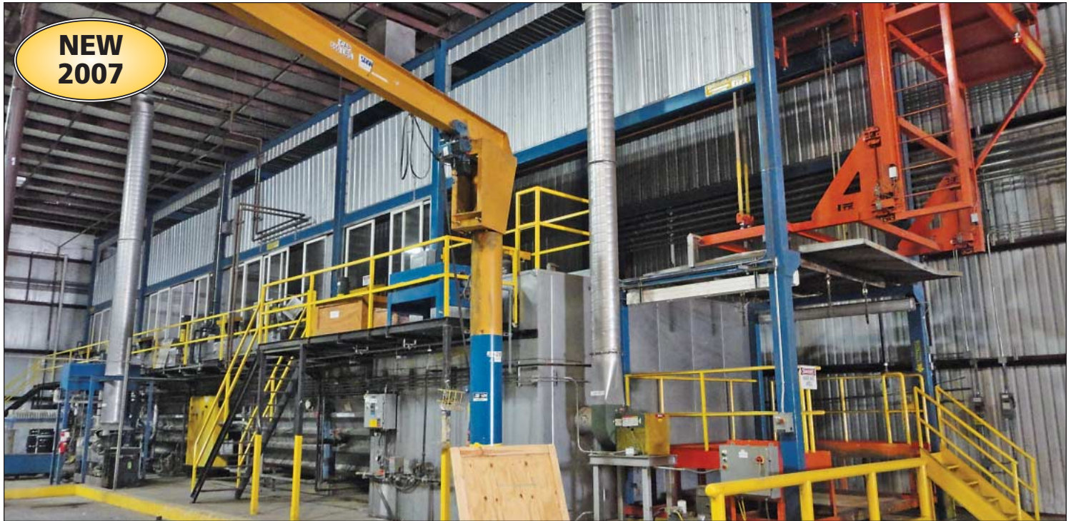
Therma-Tron-X 7-Tank Large Part Automatic Steel Phosphate Line
