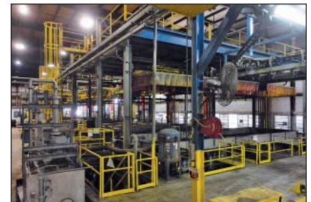
Large E-Coat Line w/ (12) 35' X 10' X 8' Tanks
