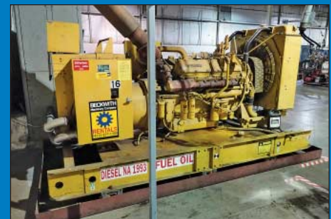
569 KVA / 455 KW Caterpillar Diesel Powered Stand-By Power Generator Set
