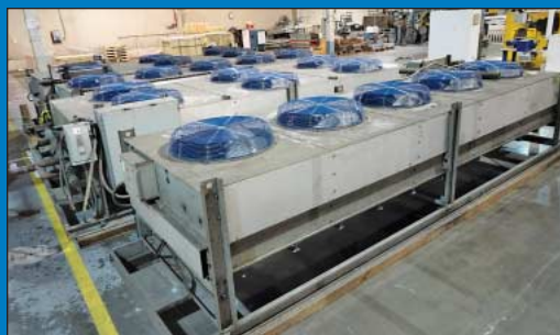
(4) Five and Six Fan Hiross Chillers
