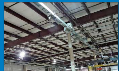
Approx. 1,100' of Copper Buss Duct
