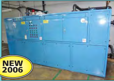
100 Ton Thermal Care Model Chill Pac CP-100X Central Chiller System w/ Condenser Units
