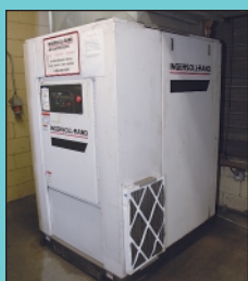
50 HP Ingersoll Rand Model SSR-EP50SE Rotary Screw Cabinet Enclosed Air Compressor
