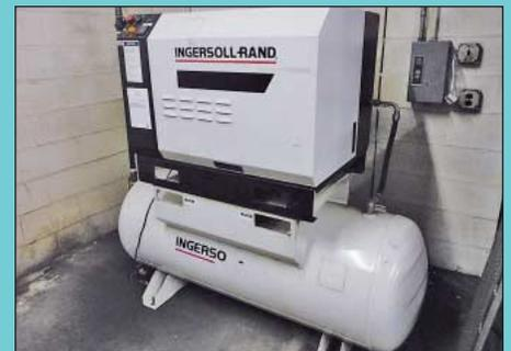
15 HP Ingersoll Rand Horizontal Tank Mounted Air Compressor
