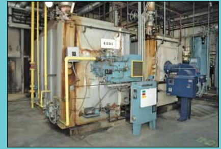
(2) International Boiler Works Model TJHC-12.5 Natural Gas Fired Hot Oil Boilers
