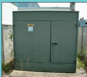
4,000 KVA Electric Supply Company Transformer
