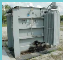
3,750 KVA Square D Three Phase Transformer
