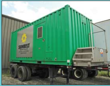
500 KW Marathon Electric Magna Max Model 572RSL4027 Diesel Power Portable Generator Set
