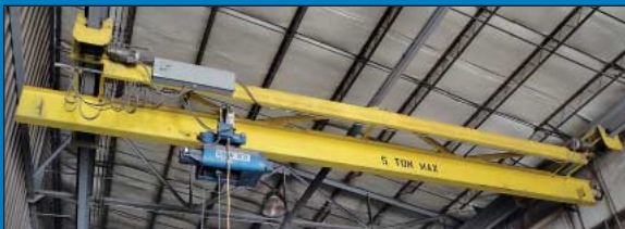
5 Ton X 25' Approx. Span Double Girder Under Hung Bridge Crane
