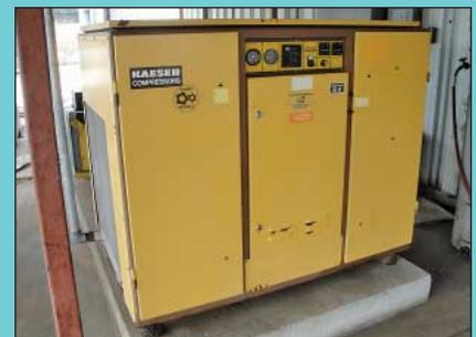
40 HP Kaeser Model BS-50 Rotary Screw Cabinet Enclosed Air Compressor
