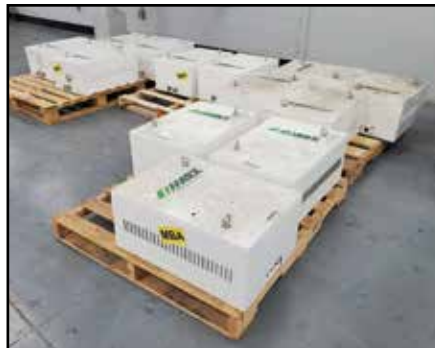
(13) MARX 55 KVA Transformers
