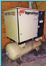
20 HP Ingersoll Rand Model SSR UP6-20-125 Horizontal Tank Rotary Screw Air Compressor
